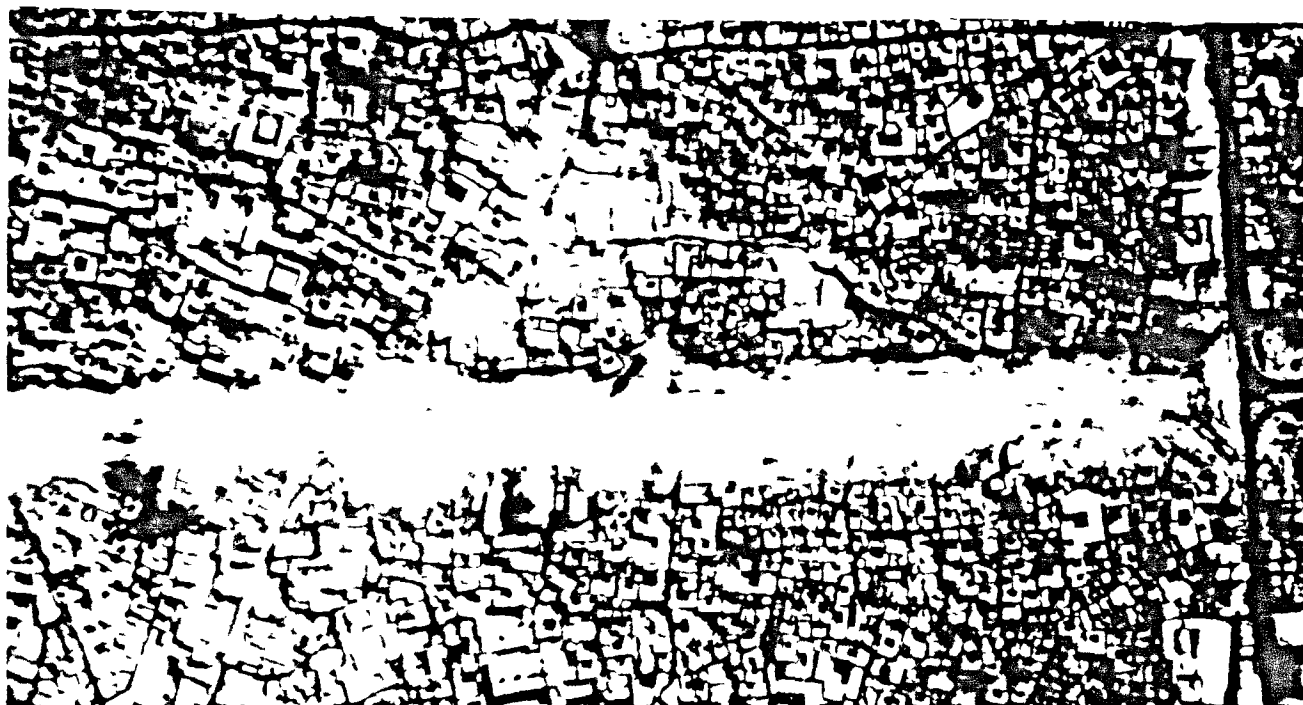
B. Aerial Photograph of Jumhuriya Street during Clearance Operations
